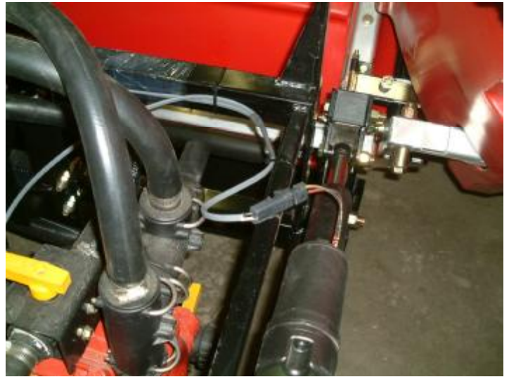
Figure 26: Slack in wire from frame to actuator
