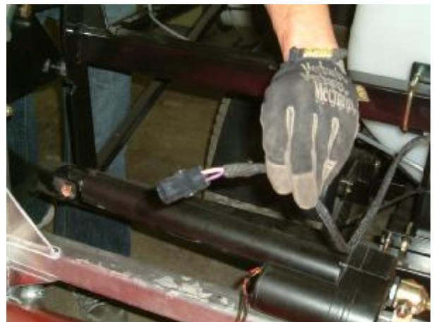
Figure 4: Installed Weather-Pak end
