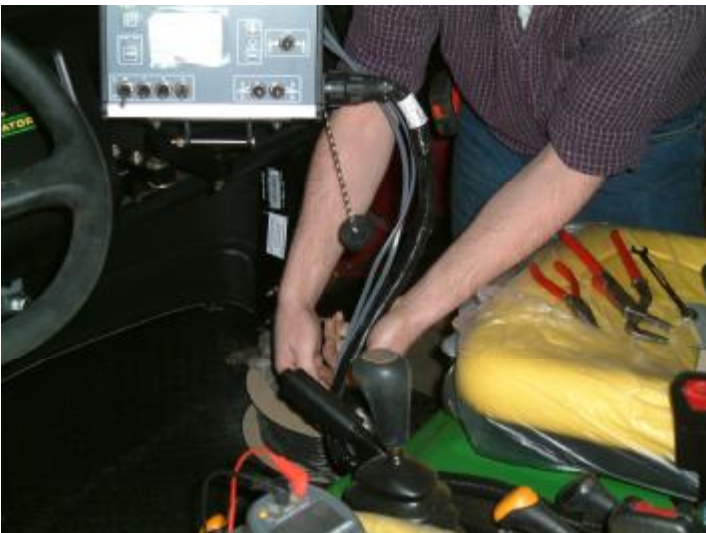
Figure 23: Taping center switch box wires to first part of existing main console wiring harness
